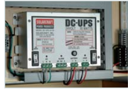
▲ The Solarcraft DC-UPS is available in 30W, 70W, and 100W, and can be paralleled for greater output.
