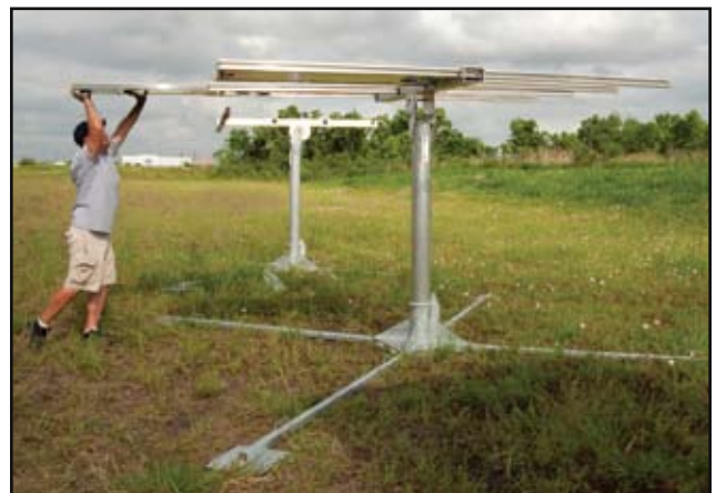
▲ Aluminum encased solar panels slide into channels on horizontal rails.
